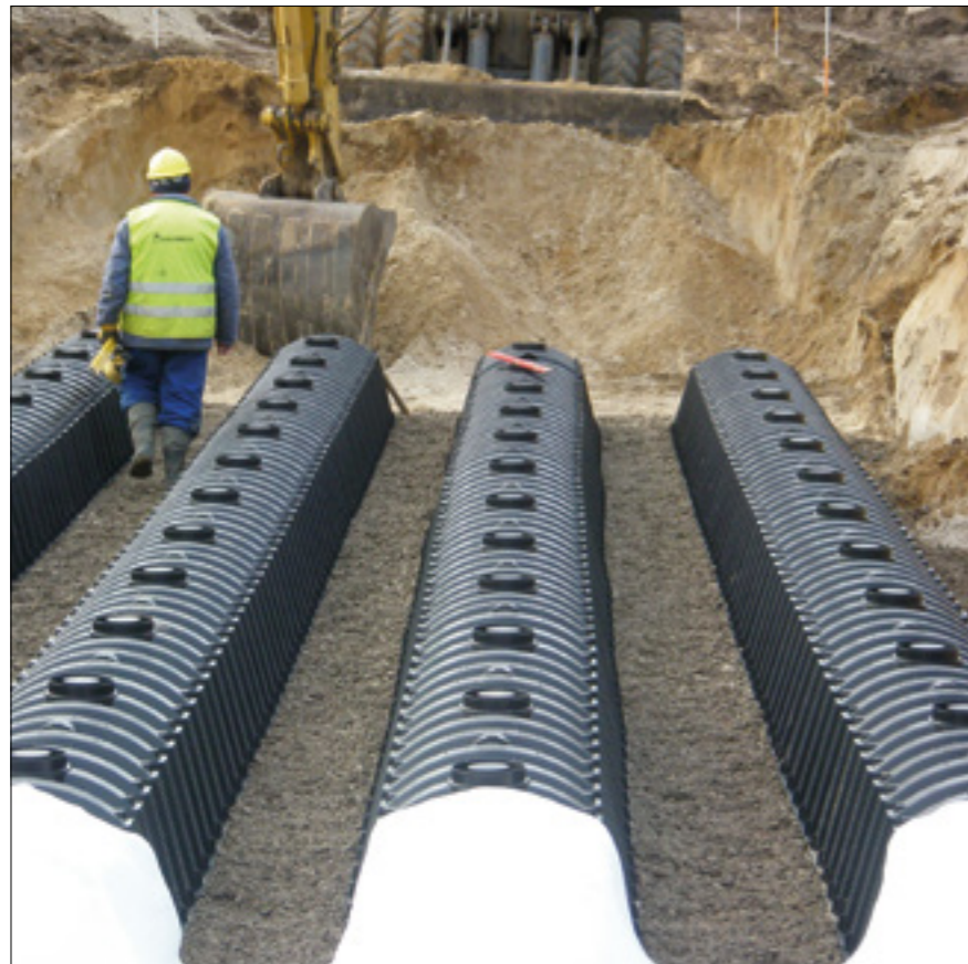
Industrial warehouse, Raben (PL)
