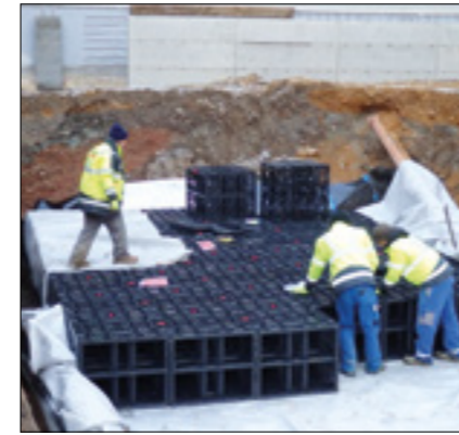
Industrial building, Tumeltsham (AT)
